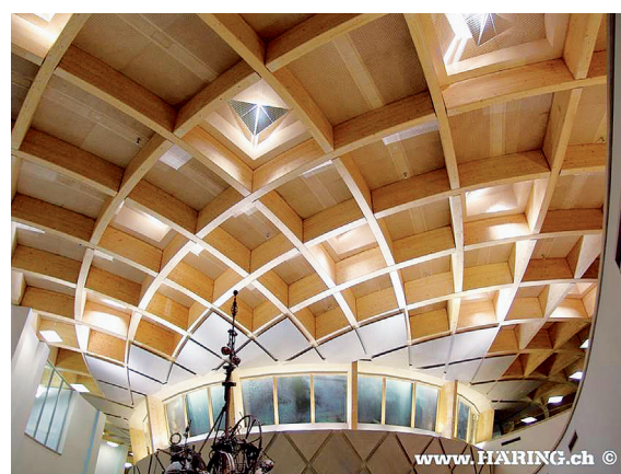
Figure 24. Salt warehouse constructed with engineered lumber ( http://www.haring.ch ).
